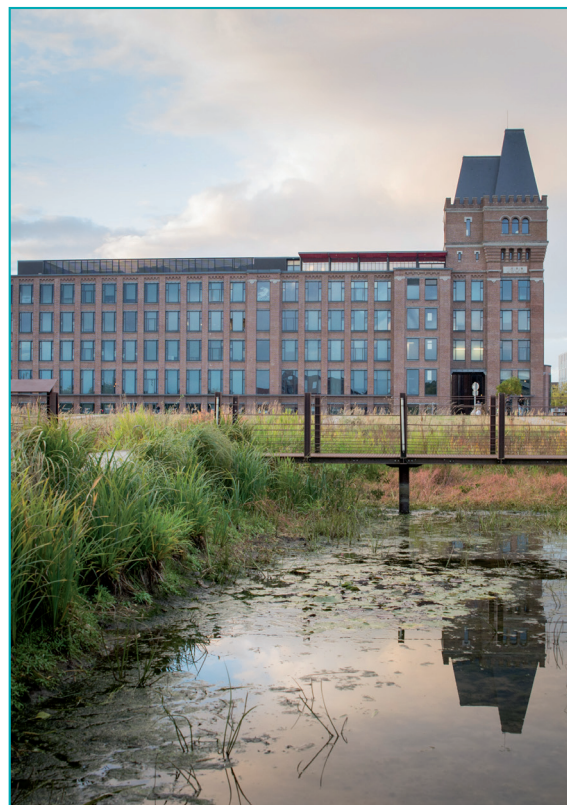
Leblan Lafont, old cotton and linen factory, today headquarters of the “site of excellence” dedicated to new technologies
